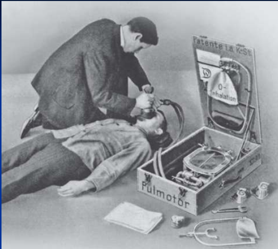
The Drager Pulmotor 1911 “Artificial Breathing Device”
